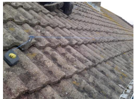
Picture showing the levelling of the roof anchors.
