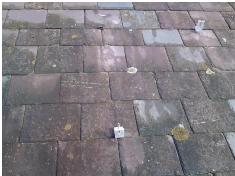
Picture showing the finished look of the Roof Bolt and anchors.
