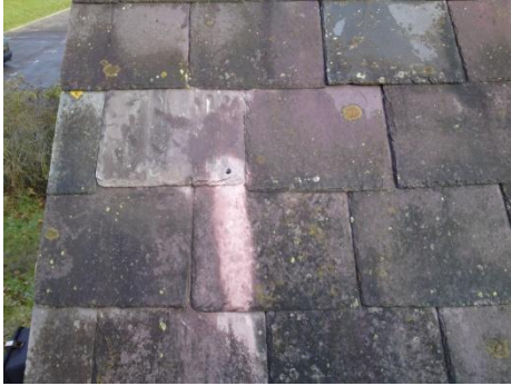
Picture showing the Slate being Drilled directly above the rafter.
