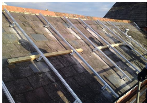
Picture showing the finished rails levelled and roof anchors sealed.
